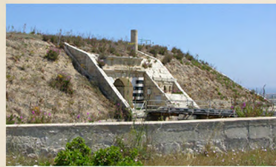
Detail of keep of Fort Mosta, showing exterior slope of earthen parapet with gateway and its small flanking musketry gallery (image source: http://www.militaryarchitecture.com/index.php/Fortifications/fort-mosta.html )
