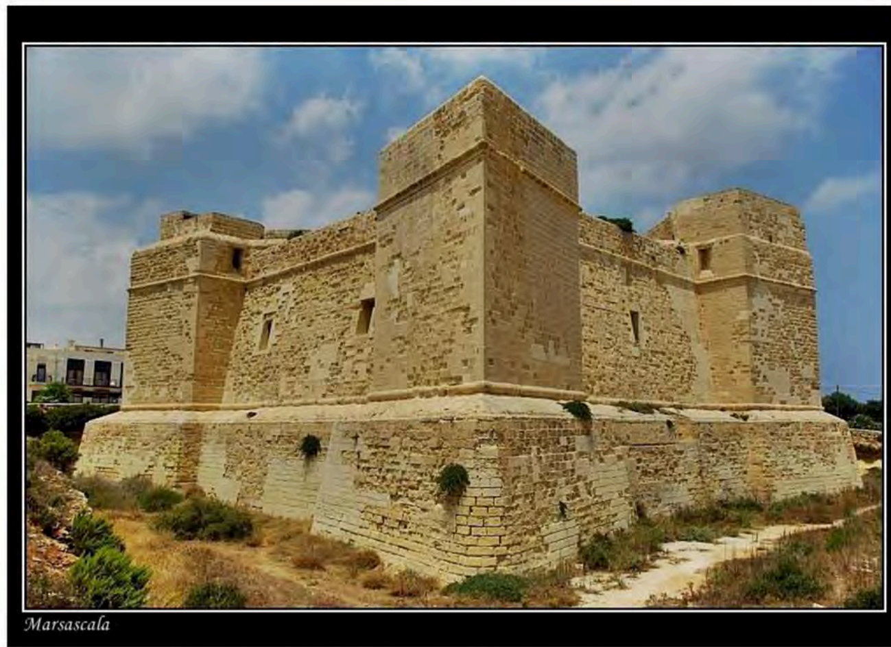
View from the northeast of St. Thomas Tower
