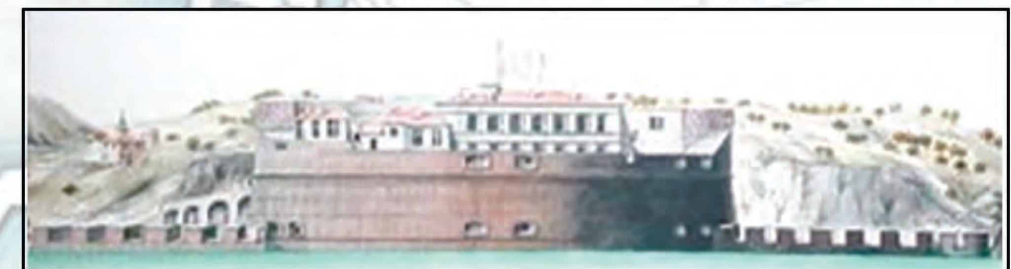
ELEVATION OF THE ROYAL TOWER SHOWS EMBRASURES ON THE TOP OF THE TOWER, SURROUNDING PROJECTIONS AND WIDE PORTS LOWER DOWN ALL DESIGNED TO FIRE GUNS AND AMMUNITION
