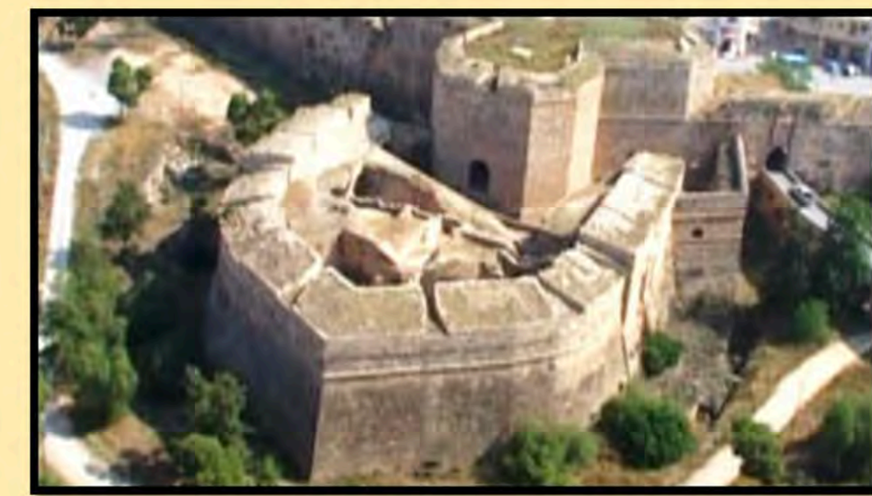
The land gate (Akkule, Ravelin, or Rivettina Bastion), Famagusta city walls, Cyprus (northern) http://www.whatson-northcyprus.com/interest/famagusta/famagusta/land_gate.htm
