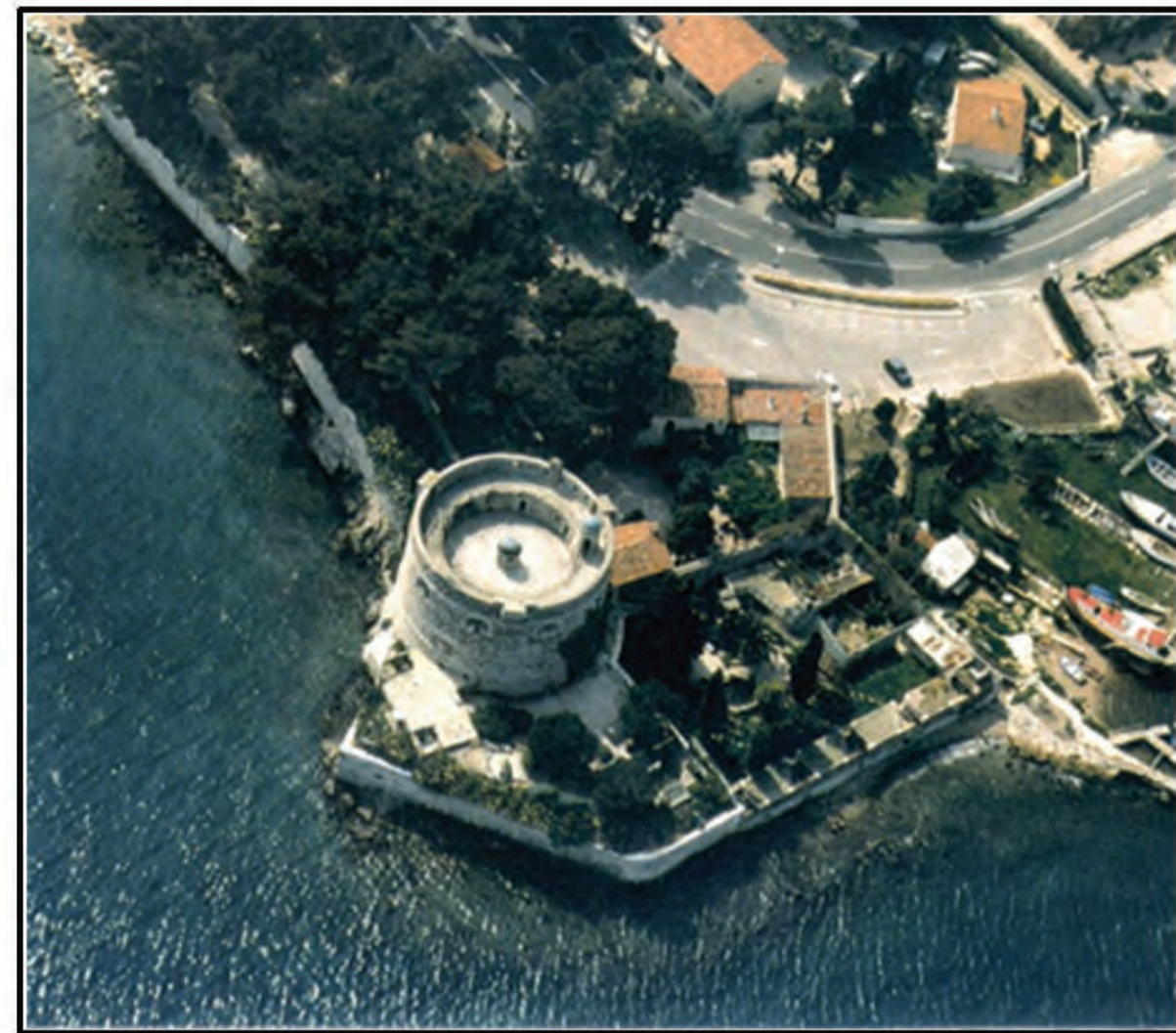
TOUR ROYALE STRATEGICALLY BUILT ON A CAPE AT THE ENTRANCE OF THE HARBOR TO FIRE AT ENEMIES COMING FROM THE SEA
