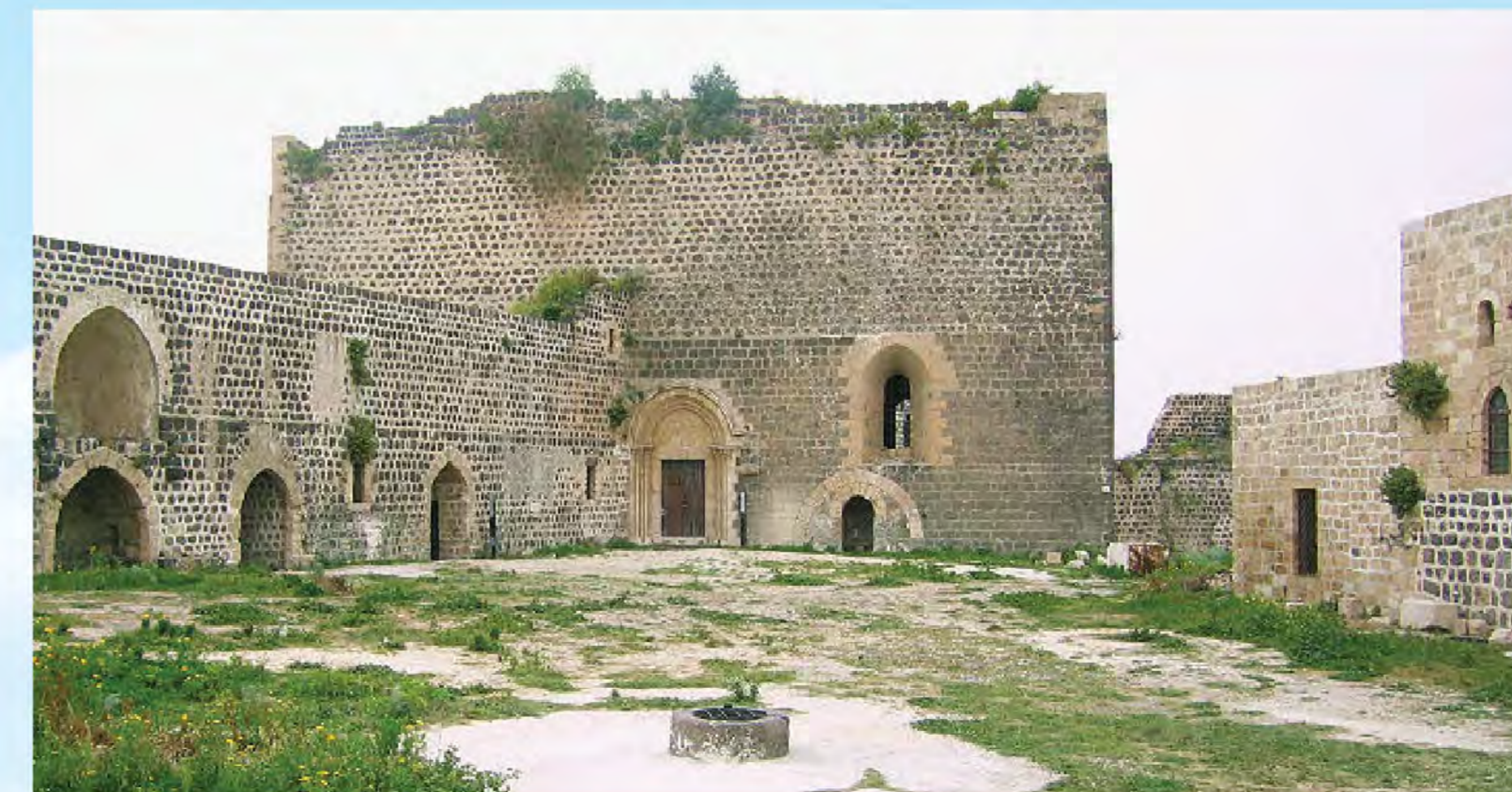
Main courtyard (chapel and hall).
